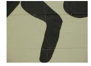
6. #60 Main Building - H-Wing Floor Cracking Repairs - \$10,000.00 Crack in the Terrazzo floor, caused by building movement, needs to be repaired.
