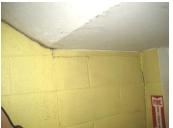
5. #45 Main Building - Large Gym Crack Repairs and Painting Walls - \$21,000.00 Large cracks in the original 1989 gymnasium wall mortar joints and through the concrete masonry units caused by building movement. Repairs will be required to prevent further deterioration. Walls and beams need to be patched and painted.
